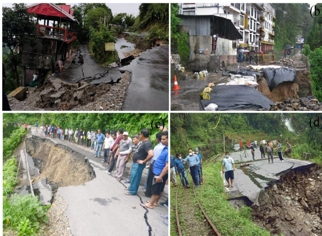
Fig. 5: Damaged roads due to landslides; a) Sukhia (Source: India.com); b) Kurseong (Source: India.com); c) and d) Gayabari (Source: The Economic Times).
